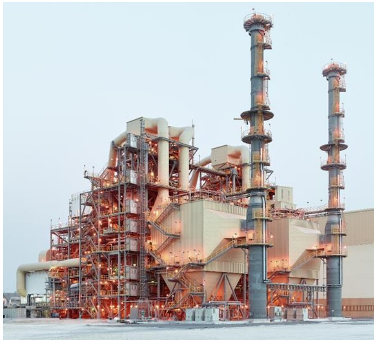
Figure 7. Two generation 5 CFB alumina calcination units.
